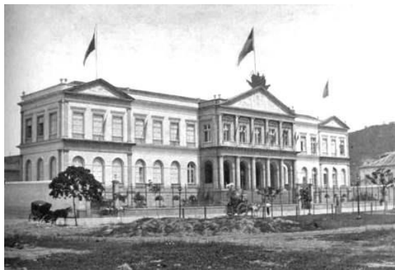
Brazilian Mint headquarters in Rio de Janeiro, from 1868 to 1984. Currently it hosts the National Archives.
